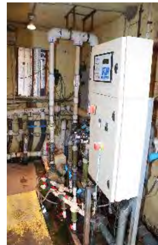
Figure 6.4 Irrigation pumps and fertilizer injector.
