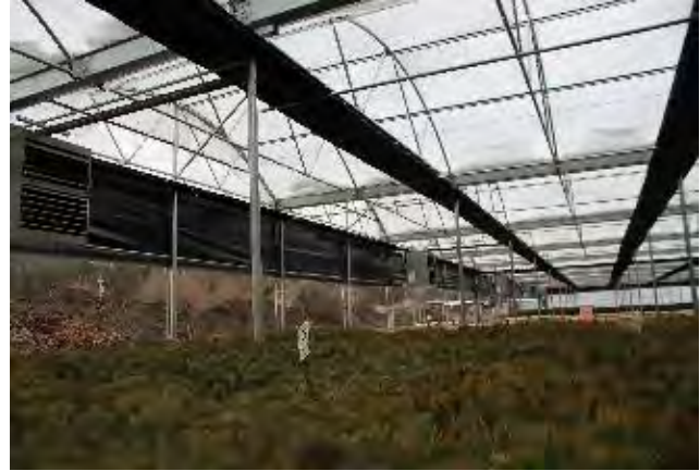
Figure 6.3 A double-layer polyethylene gutter-connected greenhouse designed to grow tree seedlings in California. Note the roll-up walls and the black-cloth system for dormancy induction using shortened photoperiod. There are also lights to extend the photo period.
